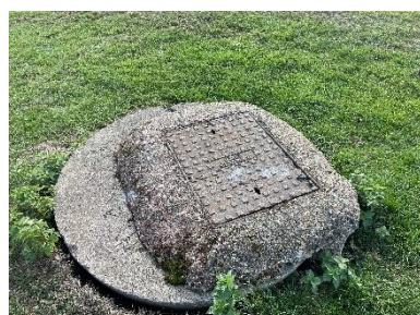
Raised concrete inspection cover
